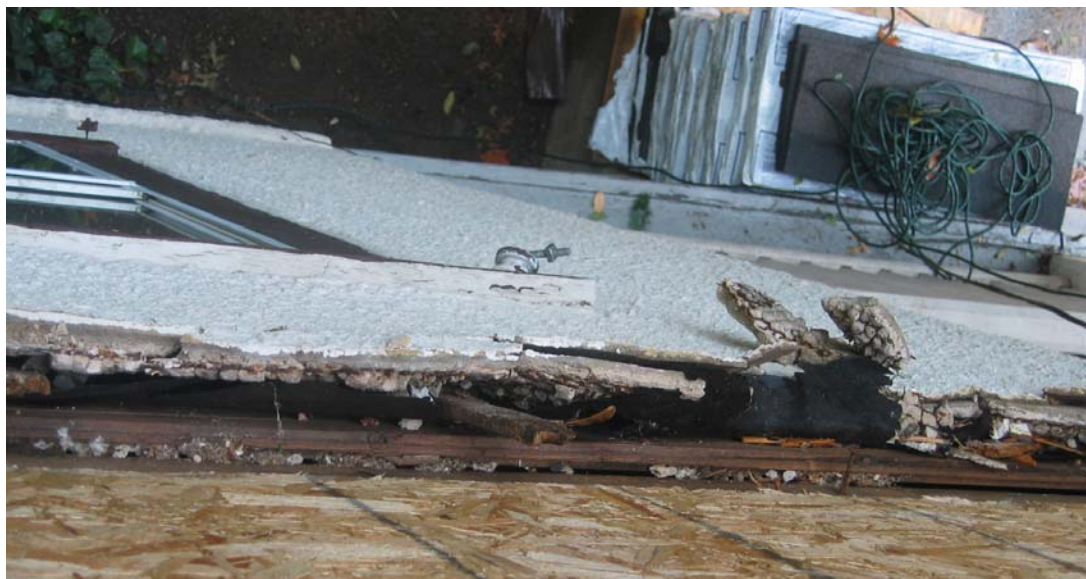
October 28, 2008 – Water seepage through exposed seams between first and second floors (42 Maple Ave.) Top – living room; above – North elevation; below – South elevation.
